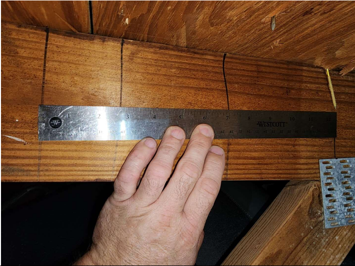
8d nails proper spacing
