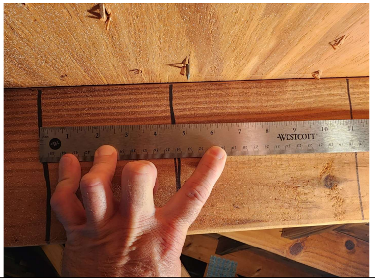
8d nails proper spacing
