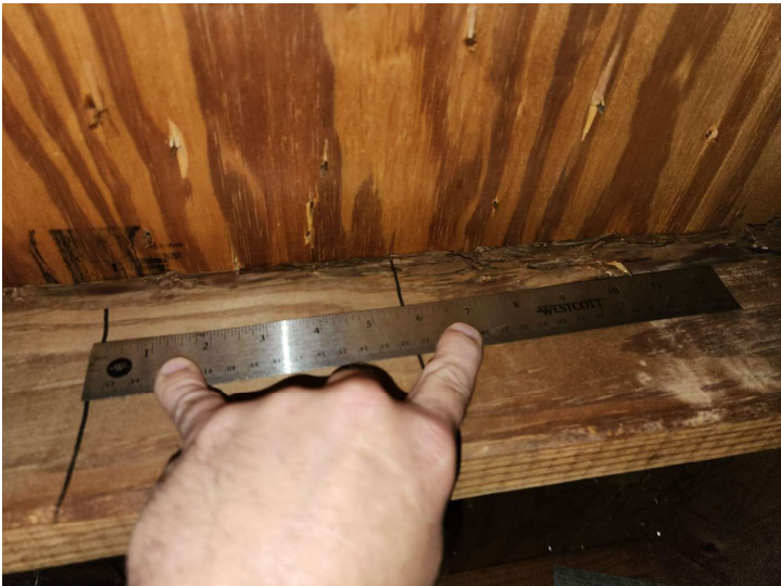
8d nails proper spacing
