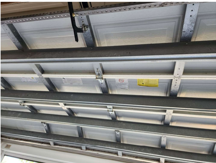
Opening Protection - Unverified
