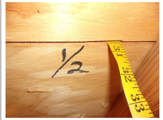
ROOF DECK THICKNESS – ½ inch plywood
