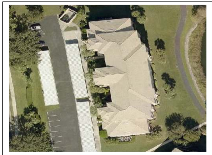
ROOF GEOMETRY – Aerial view of the hip roof shape
