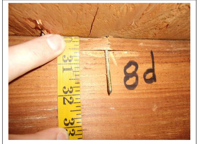
ROOF DECK ATTACHEMNT – 8d ring shank nails added in 2021
