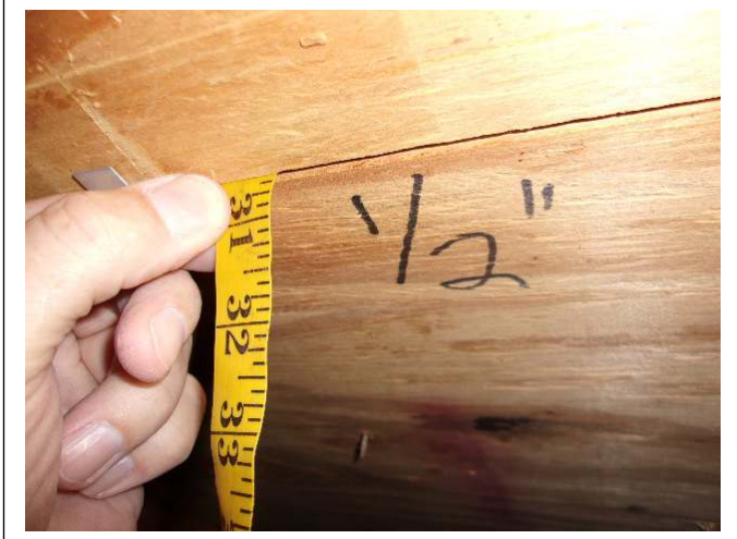
ROOF DECK THICKNESS – ½ inch plywood
