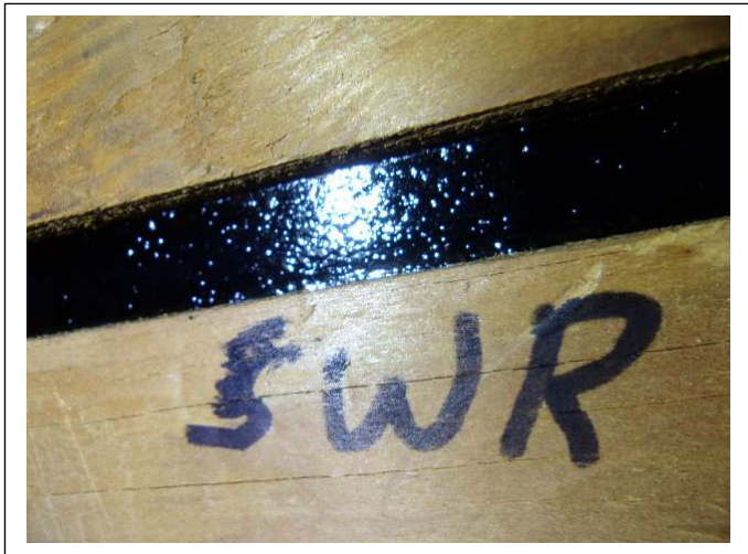
SECONDARY WATER BARRIER – A polymer adhesive (peel & stick) SWR Barrier was installed on the entire roof deck in 2021
