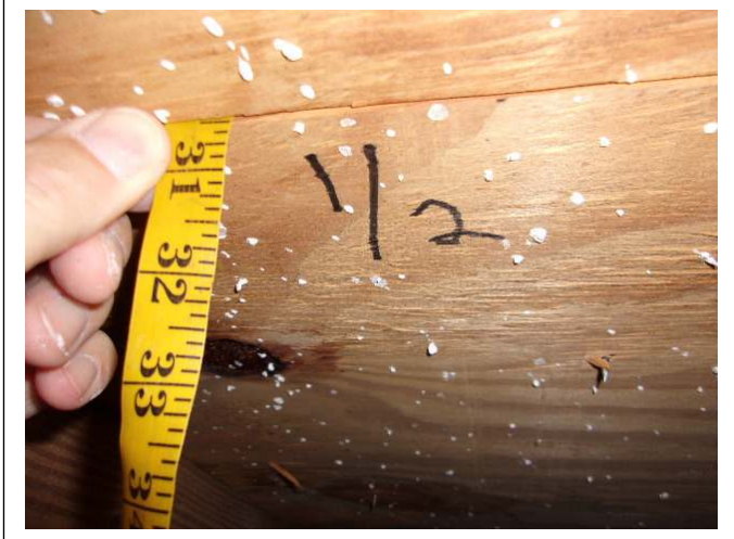
ROOF DECK THICKNESS – ½ inch plywood
