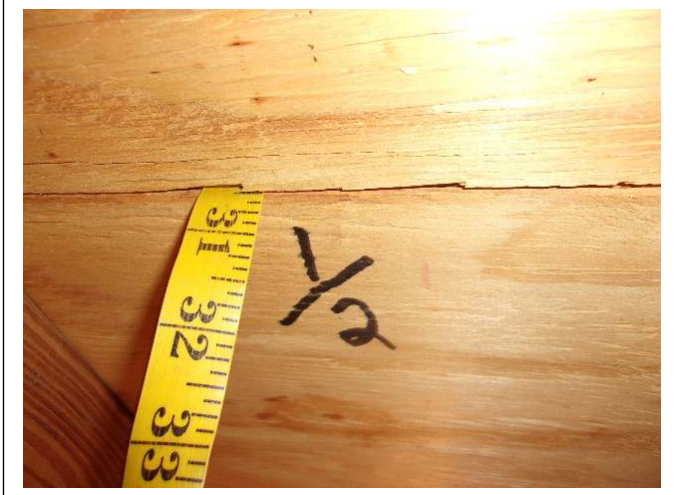
ROOF DECK THICKNESS – 1/2 inch plywood
