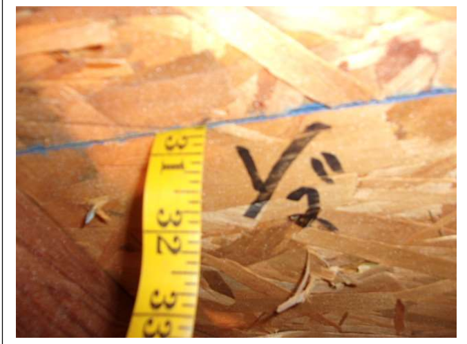
ROOF DECK THICKNESS – ½ inch OSB
