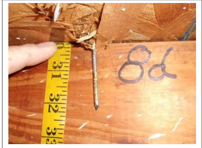
ROOF DECK ATTACHEMNT – 8d ring shank nails installed in 2018
