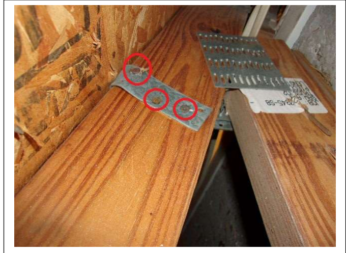
ROOF TO WALL ATTACHMENT – Properly installed Single Wraps
