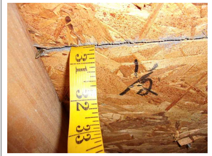
ROOF DECK THICKNESS – ½ inch OSB
