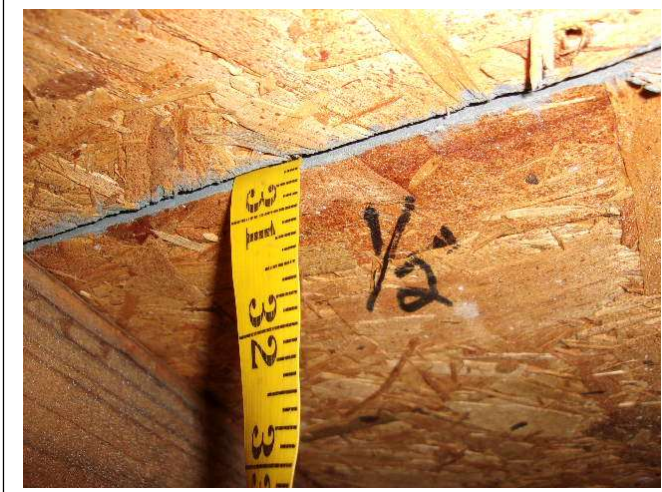
ROOF DECK THICKNESS – ½ inch OSB
