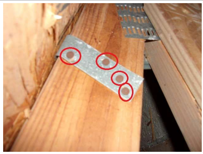
ROOF TO WALL ATTACHMENT – Properly installed Single Wraps
