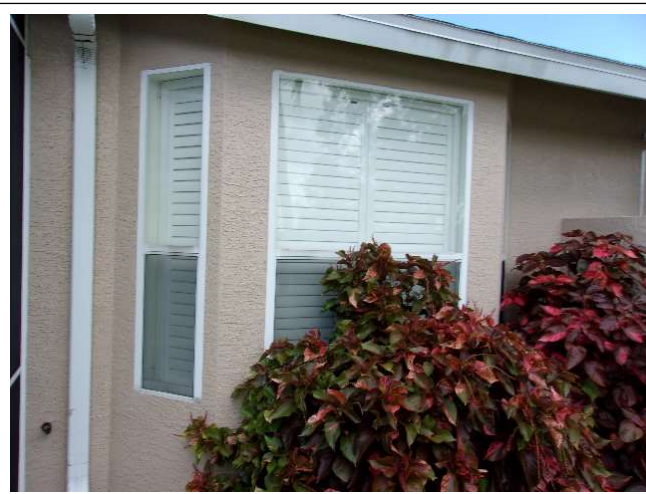
OPENING PROTECTION – Although some unit owners have installed wind-borne debris protection devices, others have not, leaving some openings (entry doors, window units and/or sliding doors) unprotected
