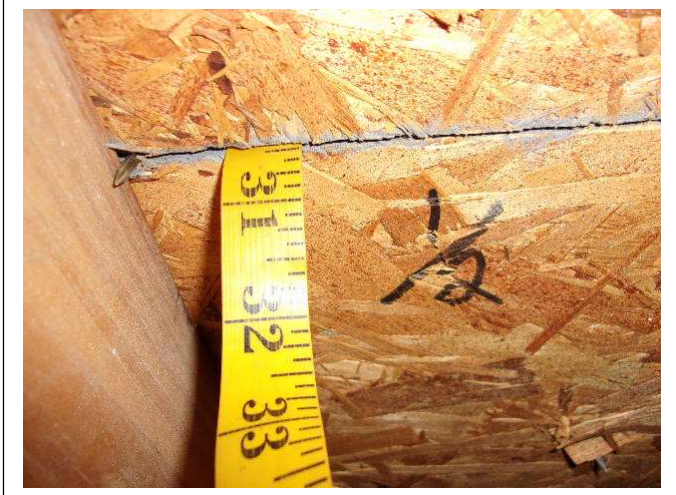
ROOF DECK THICKNESS – ½ inch OSB
