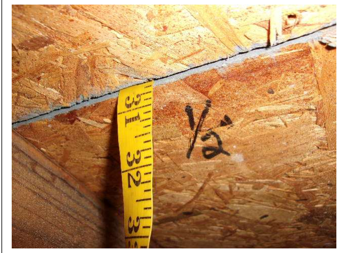
ROOF DECK THICKNESS – ½ inch OSB
