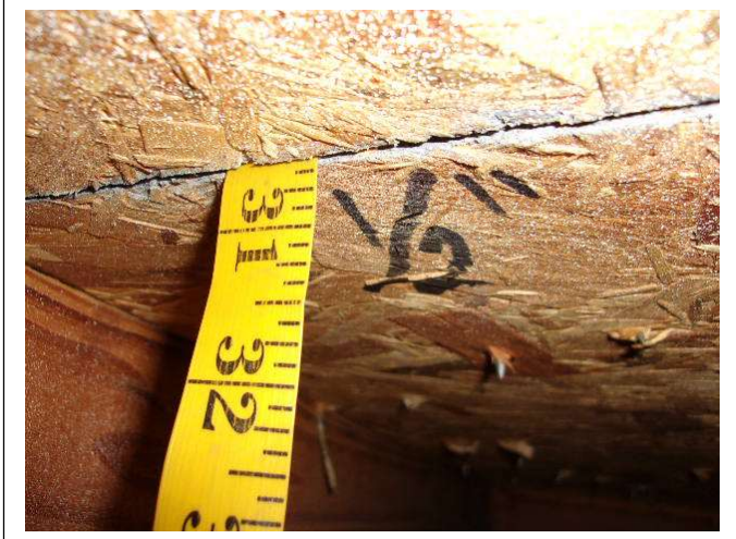
ROOF DECK THICKNESS – ¾ inch OSB
