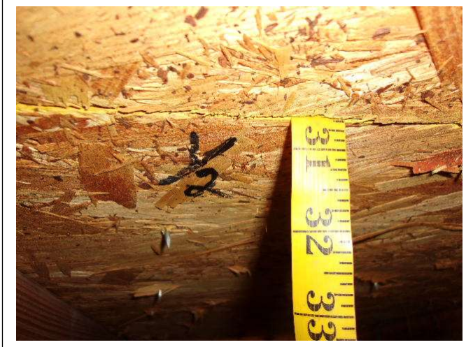
ROOF DECK THICKNESS – ½ inch OSB
