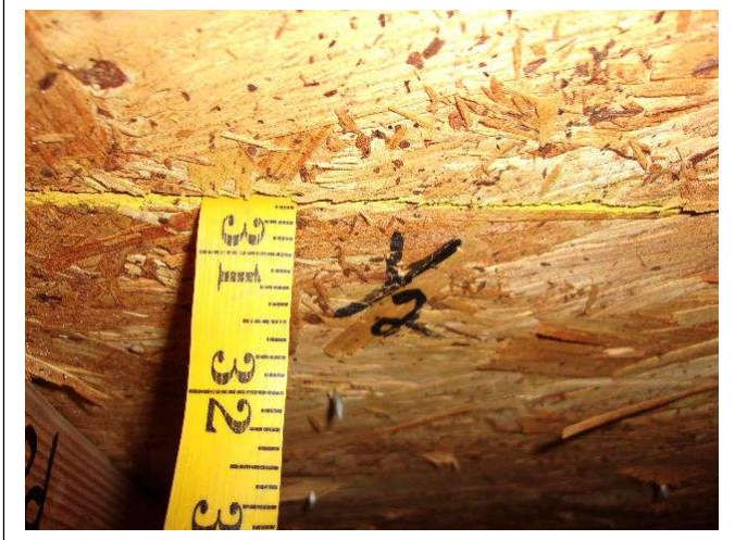
ROOF DECK THICKNESS – ½ inch OSB
