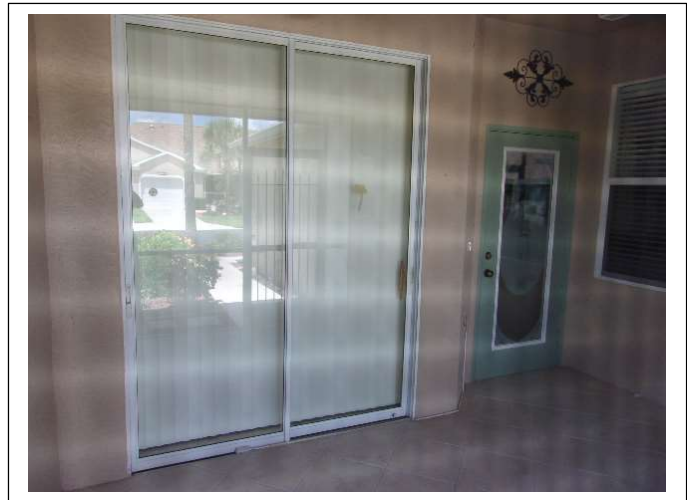
OPENING PROTECTION – Although some unit owners have installed wind-borne debris protection devices, others have not, leaving some openings (entry doors, window units and/or sliding doors) unprotected
