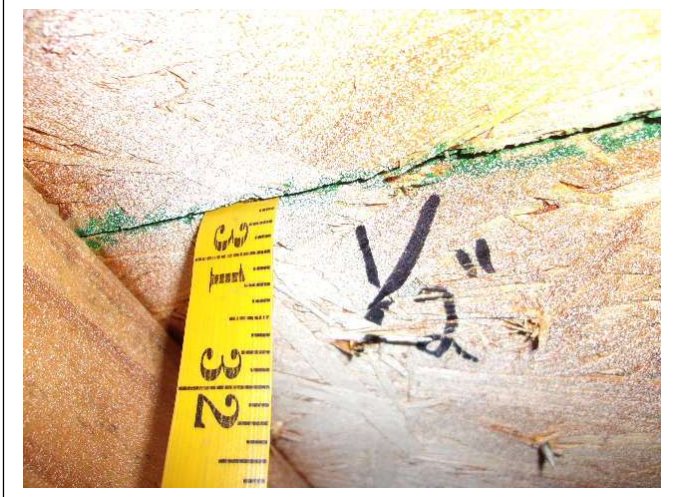
ROOF DECK THICKNESS – ½ inch OSB
