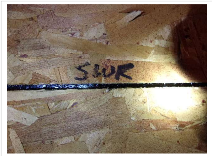
SECONDARY WATER BARRIER – A polymer adhesive (peel & stick) SWR Barrier was installed on the entire roof deck in 2018
