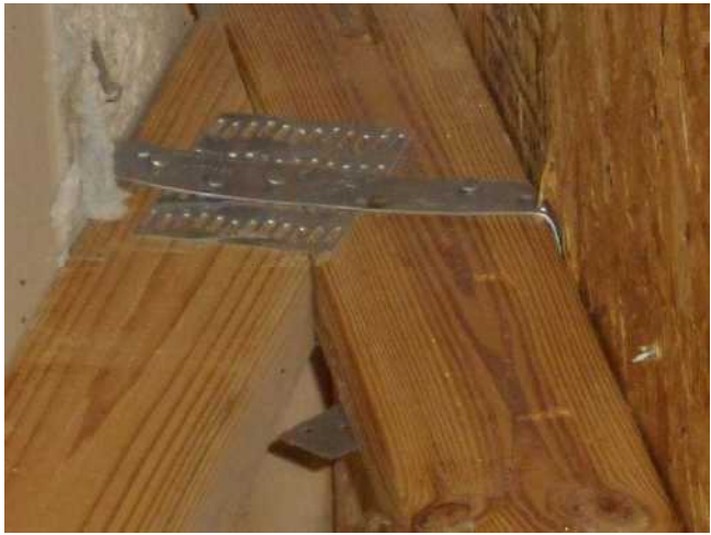
ROOF TO WALL ATTACHMENT
