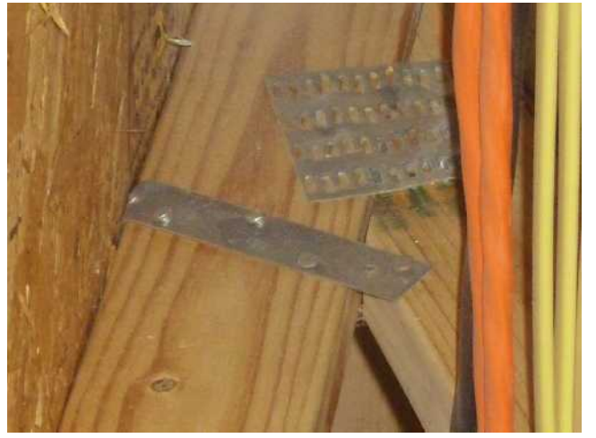
ROOF TO WALL ATTACHMENT
