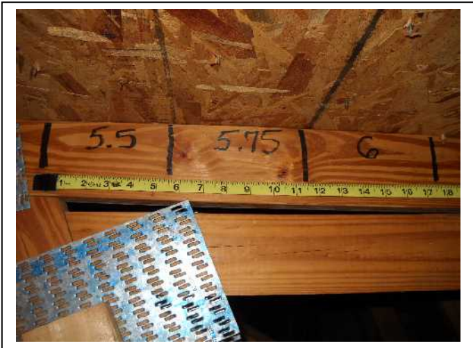
ROOF DECK ATTACHMENT
