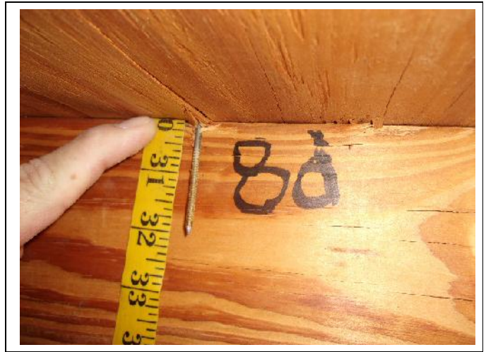
ROOF DECK ATTACHMENT – 8d ring shank nails added in 2017
