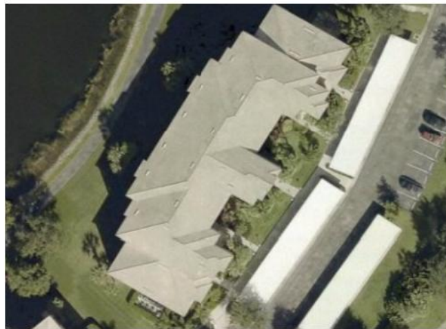
ROOF GEOMETRY Aerial View of the Ilip Roof Shape
