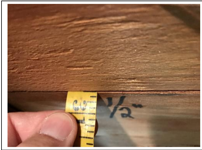
ROOF DECK THICKNESS – ½ inch plywood
