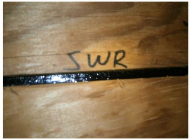
SECONDARY WATER RESISTANCE A polymer adhesive "peel & stick" SWR Barrier was installed on the entire roof deck in 2017
