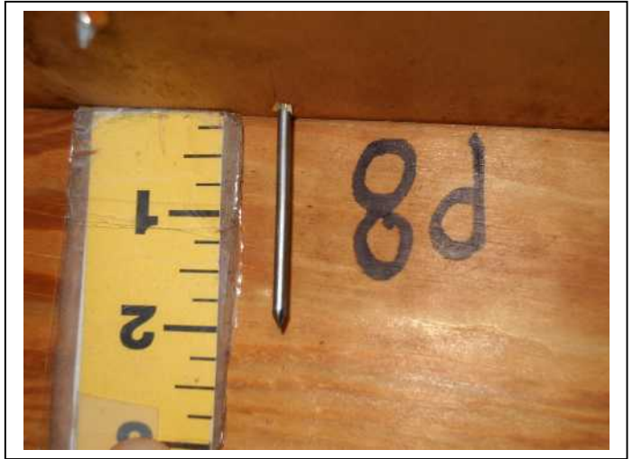
ROOF DECK ATTACHMENT
