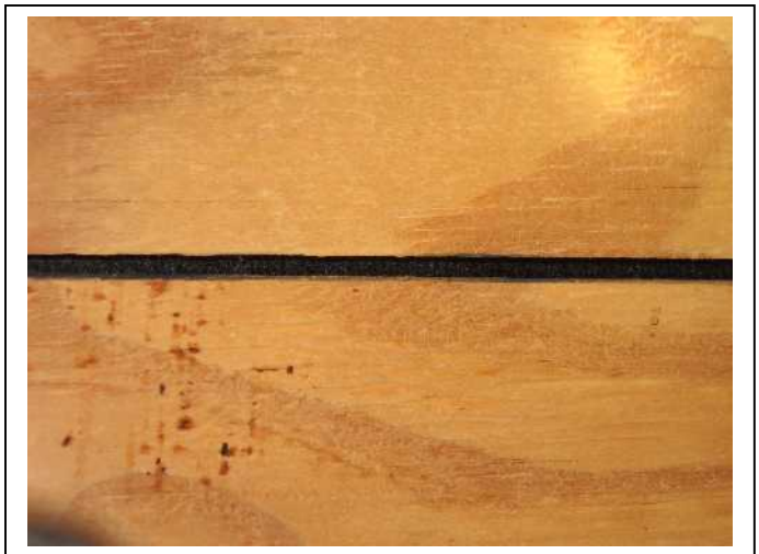
SECONDARY WATER BARRIER – Is not present.
