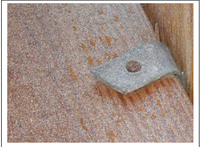
ROOF TO WALL ATTACHMENT
