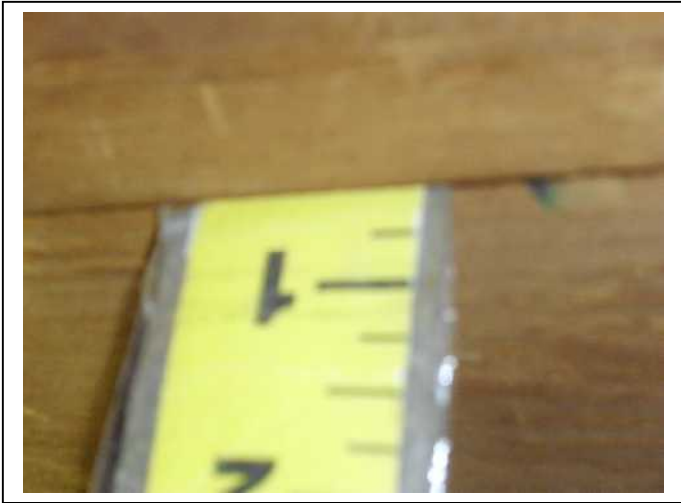
ROOF DECK THICKNESS
