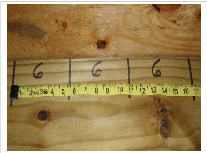
ROOF DECK ATTACHMENT
