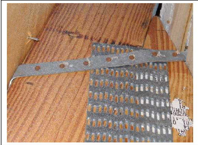
ROOF TO WALL ATTACHMENT
