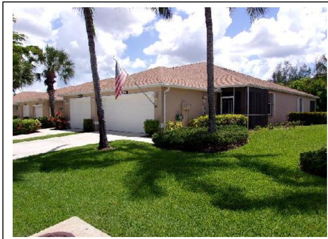
ROOF GEOMETRY – Hip Roof Shape
