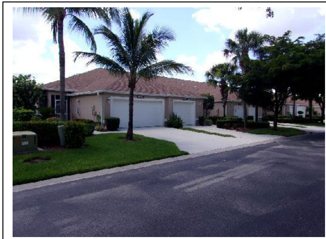
ROOF GEOMETRY – Hip Roof Shape
