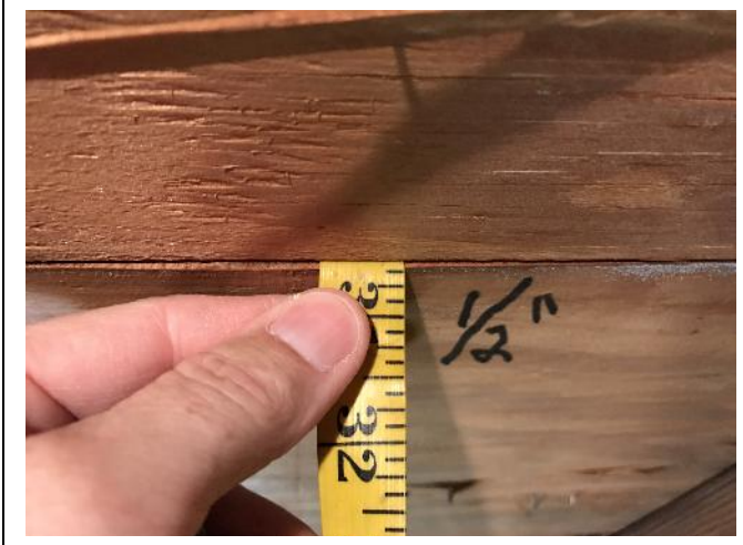
ROOF DECK THICKNESS – ½ inch plywood
