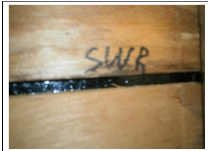
SECONDARY WATER RESISTANCE – A polymer adhesive “peel & stick” SWR Barrier was installed on the entire roof deck in 2016
