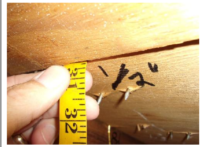
ROOF DECK THICKNESS – ½ inch plywood
